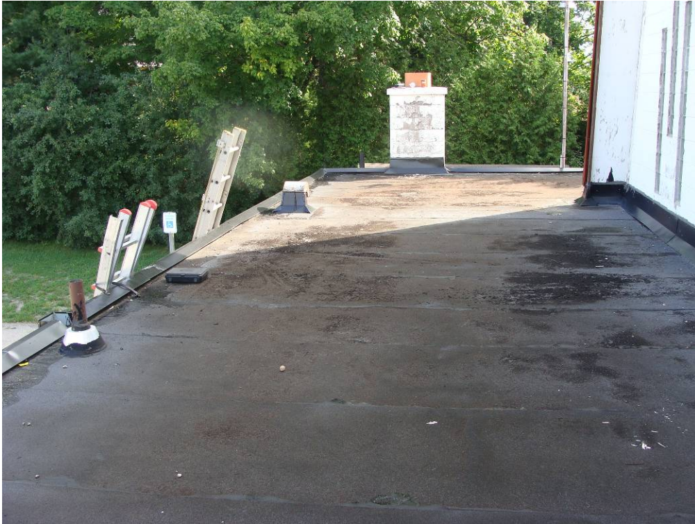
Photograph 7: View of the low roof area over the entrance foyer.
