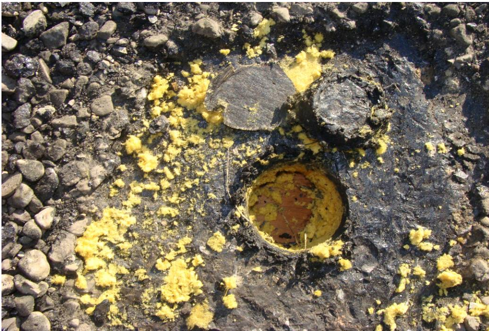
Photograph 2: View of the core cut at the main roof area.
