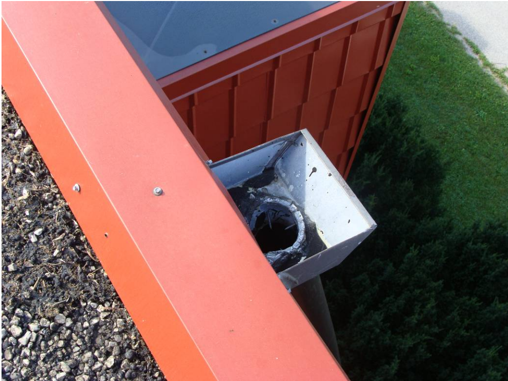
Photograph 4: View of a typical scupper drain.
