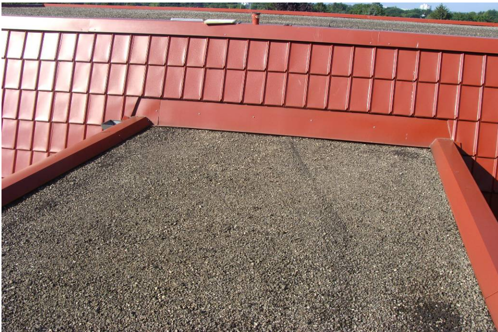
Photographs 5 and 6: View of the sacristy/choir area roof.
